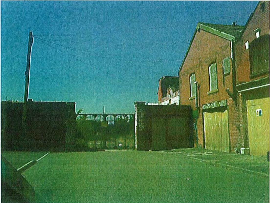
Figure 20 A view of the south eastern boundary and entrance to the site from Uxbridge Street.
