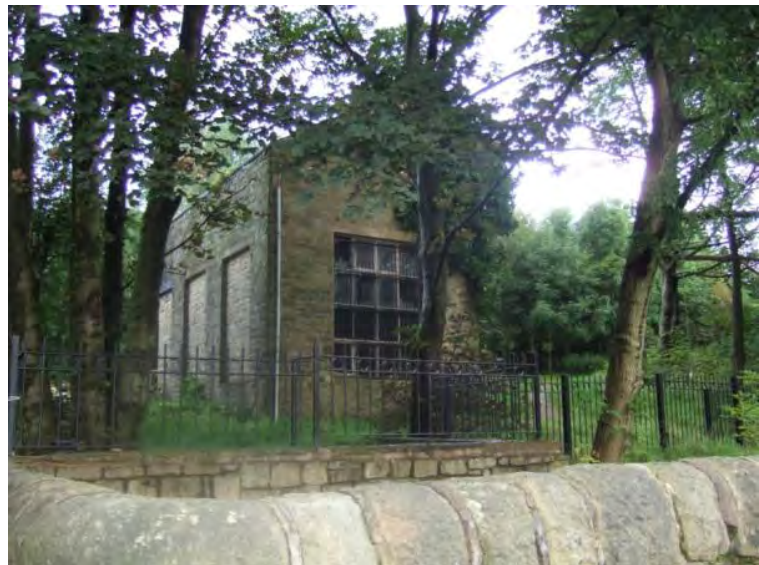
Former pump house, Castle Lane
