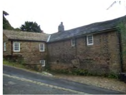
Carr House, Carr Lane (rear view)
