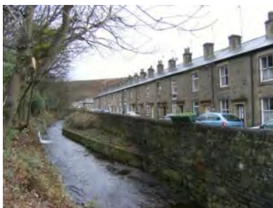
Canalised section of Carr Brook to the north of Long Row
