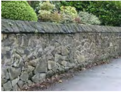
Retaining wall at Castle Terrace, Buckton Vale Road
