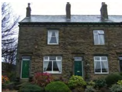
Castle Terrace: Original timber doors
