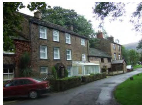
Flash Settlement, Carrbrook Road
