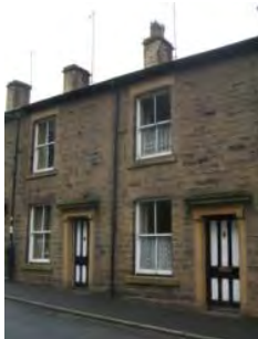
Long Row: Original timber doors and sash windows
