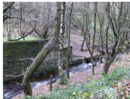
Remains of industrial water systems at Carr Brook/Staly Brook, Castle Clough
