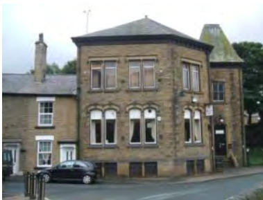
Buckton Vale Institute, Buckton Vale Road
