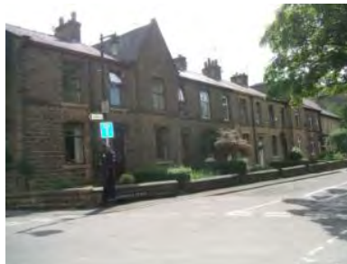
Beaconsfield Terrace, Numbers 17-29 Castle Lane
