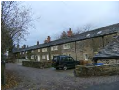
Numbers 1,2 & 3 and Moorgate Farmhouse, School Lane
