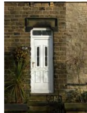
Replacement door in uPVC
