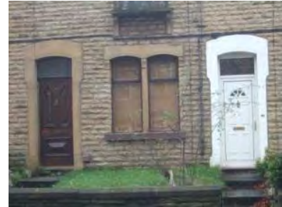
Original timber and replacement uPVC door
