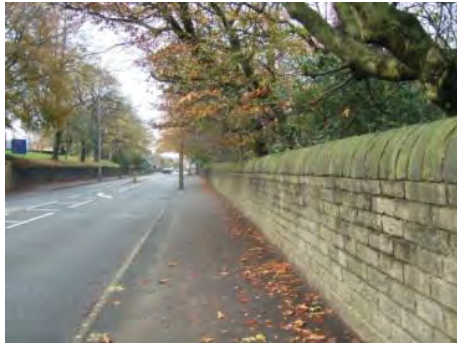
Stone retaining walls, Huddersfield Road
