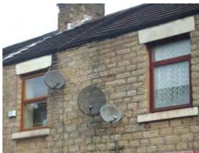
Example of satellite dishes and modern roof tiles
