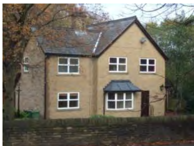
New Vicarage, Huddersfield Road
