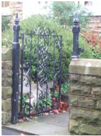
Original gate piers, Albion Crescent
