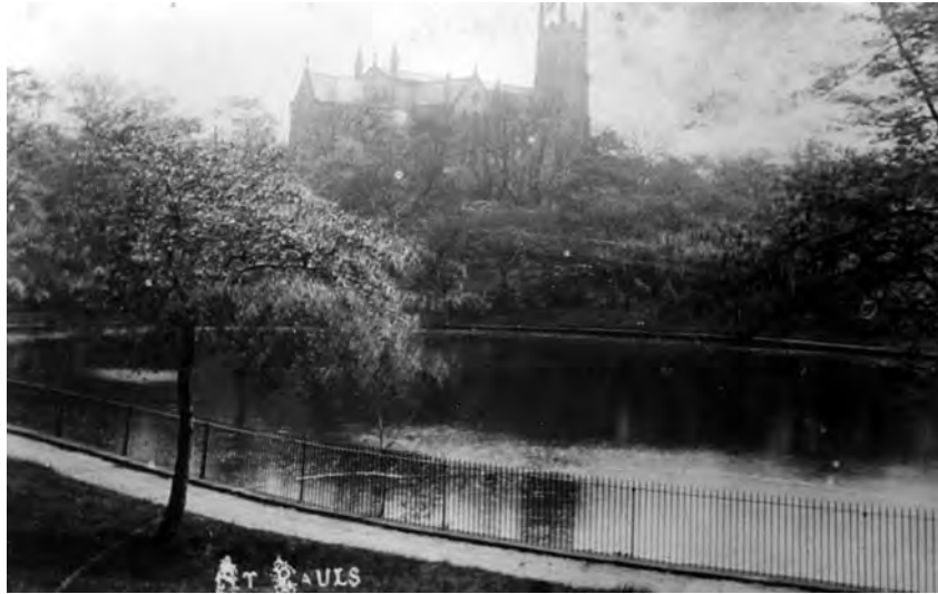
Lake at Brookfield House (the home of James Wilkinson) and St. Paul's Church c.1910. House now demolished and lake filled in between 1910 and 1933 6
