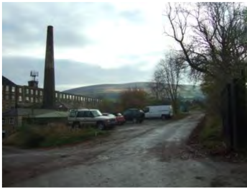
Area between Copley Mills and St. Paul's Church
