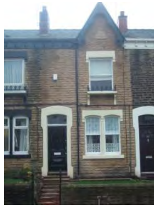
Stone name plate, cast iron detailing and original door, Albion Terrace
