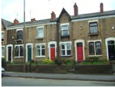
Albion Crescent, Number 78-86 Huddersfield Road
