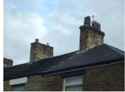
Modern replacement roof tile adjacent to original stone slate roof
