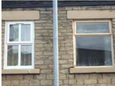
Example of replacement windows in timber and uPVC
