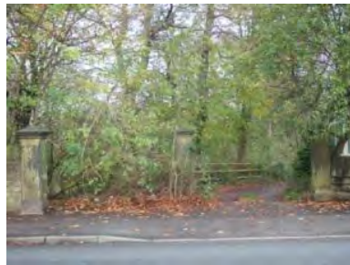
Gate piers to former Brookfield House
