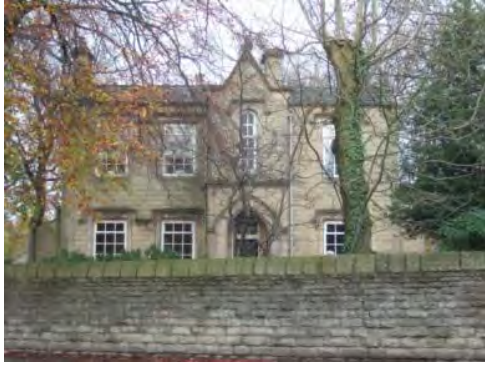
Ash Bank House
