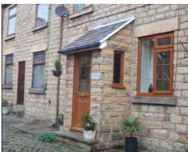
Example of an additional porch
