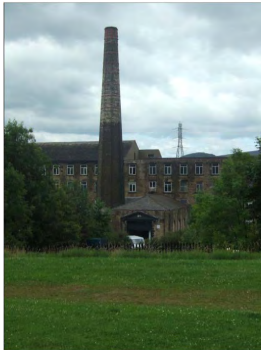
Copley Mill: former engine house and chimney
