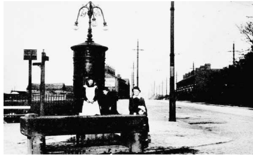
Trough and Transformer (electricity supply for trams),
