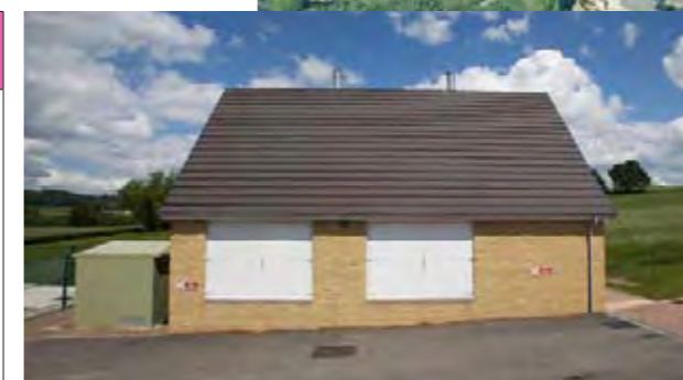
Biomass heating plant 'energy centre'
