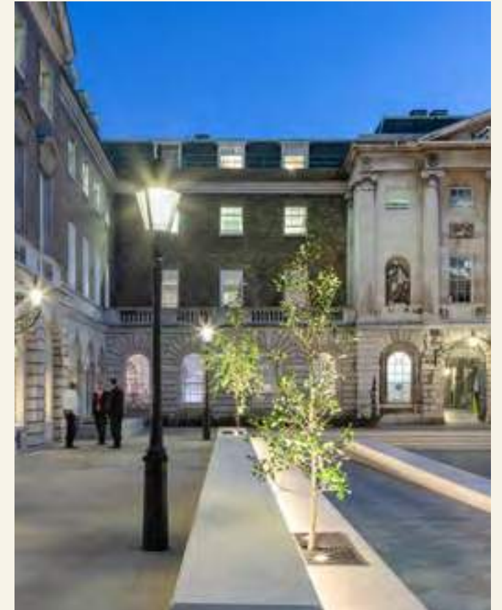
↑ Traditional style lighting and lamp posts to compliment existing character (Peter Landers Photography)
