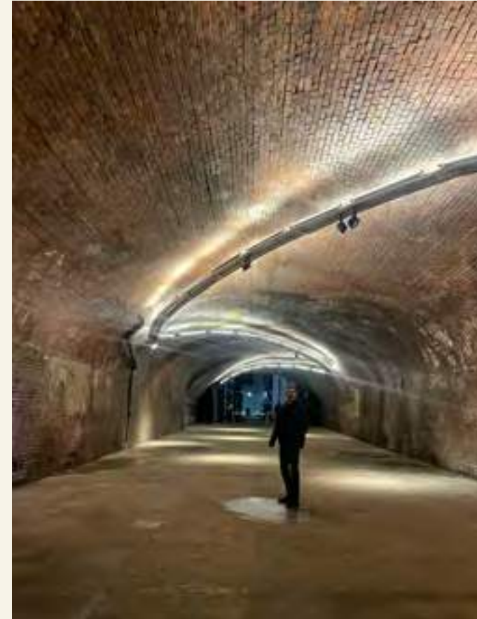
↑ Creative lighting under the bridge connecting visitors from the station to town
