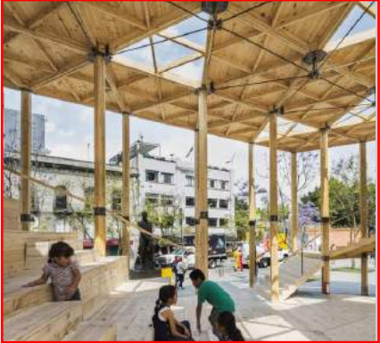
House of Switzerland Pavilion
