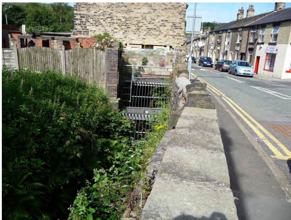
Plate 37 – Trash screen at Carr Brook culvet inlet
