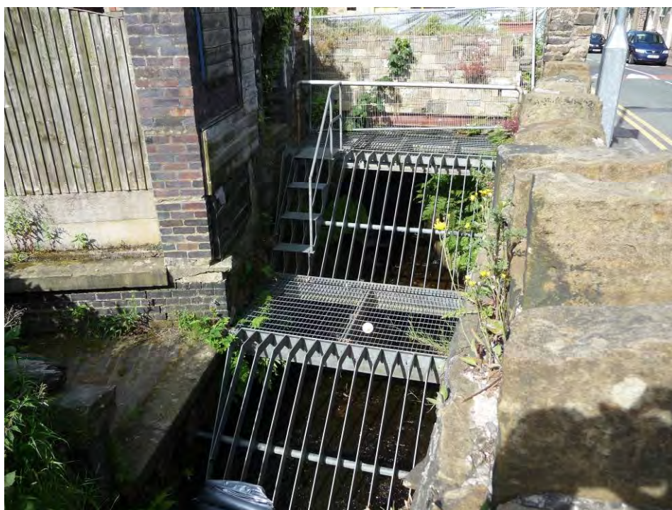
Plate 38 – Trash screen at Carr Brook culvet inlet
